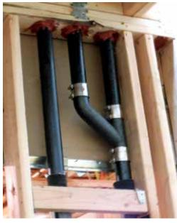
Plumbing joints with pipes nested in joint to allow for vertical movement of structure
