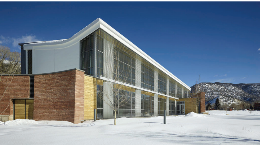
Wood is a strategy used to denote building entries and as a transition between exterior materials.
