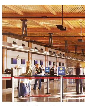
ABOVE: For the Jackson Hole Airport in Wyoming, designers chose wood because of its varied grain and color palette, as well as its ability to perform structurally under a variety of loading conditions. The inherent fire performance of heavy timber construction was vital in allowing the wood to be exposed. Winner of a 2015 WoodWorks Wood Design Award.
