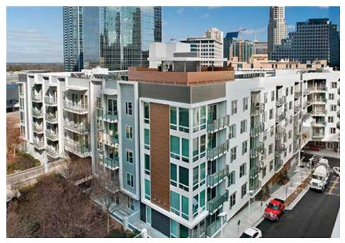
At Crescent Terminus in Atlanta, stairs are designed with double stud walls providing a 2-hour fire separation. The team specified concrete block construction at the elevator shafts, and used a wood-frame wall to separate the elevator shaft from the rest of the construction. They also filled the interstitial space between floors with blown insulation instead of using sprinklers, which avoided technical concerns related to having sprinklers in inaccessible spaces.
