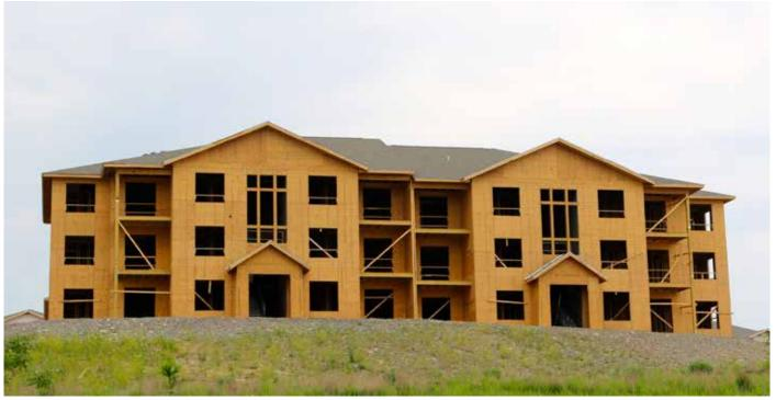
When structural panels such as plywood or oriented strand board (OSB) are properly attached to lumber floor, roof and wall framing, they form diaphragms and shear walls that are exceptional at resisting seismic forces.
