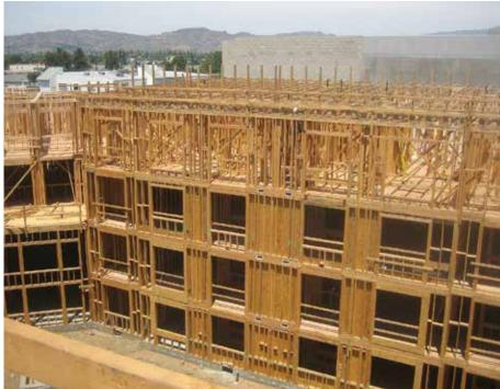
Structures with ductile detailing, redundancy and regularity are favored for seismic force resistance. This structure includes repetitive wood framing and ductile nailed wood structural panel shear walls and diaphragms.
