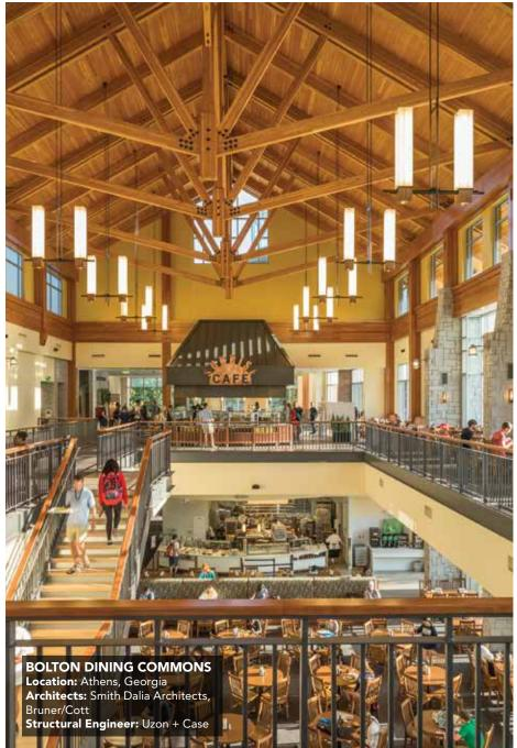
In this 55,555-square-foot dining commons at the University of Georgia, glulam trusses and Douglas-fir structural roof decking respond to the client's desire for natural materials that evoke feelings of warmth and comfort.
