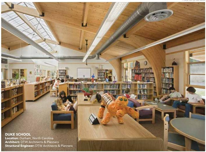
To create a welcoming environment, the Duke School library is framed with glulam arches that span the space. Between the arches are glulam beams and, above those, spanning in the opposite direction, exposed tongue and groove decking.
