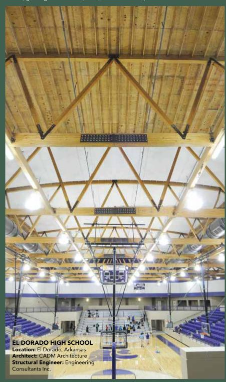
With seating for 2,200 people, this is one of the larger assembly spaces by high school standards. The roof is made from curved bowstring trusses spanning about 165 feet. Originally designed in structural steel, the switch to a bowstring truss wood roof saved the project \$60,000.
