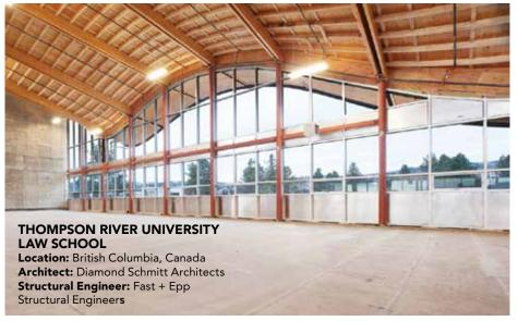
Prefabricated panels for this 400-foot-long roof at Thompson River University Law School in British Columbia were erected in roughly six weeks. The glulam frame is supported by wood purlins made from trees killed by the Mountain Pine Beetle.
