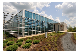
Allstate Insurance Data Center Consolidation Blade Technology / Virtualization Software Green Data Center of the Year, DeCAY Awards
