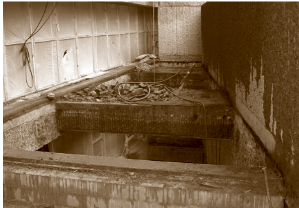
The Art + Architecture Building at Yale University. A prior renovation covered architect Paul Rudolph's light wells with a single flat roof. Such misguided "improvements" can destroy both the functionality and aesthetics of Modern-era buildings, many of which are beginning to cross the half-century mark.
