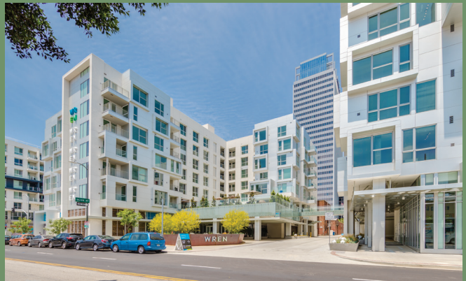
Five stories of wood construction built on a double podium enabled high densities at Wren, a new residential community designed by Togawa Smith Martin for downtown Los Angeles.
