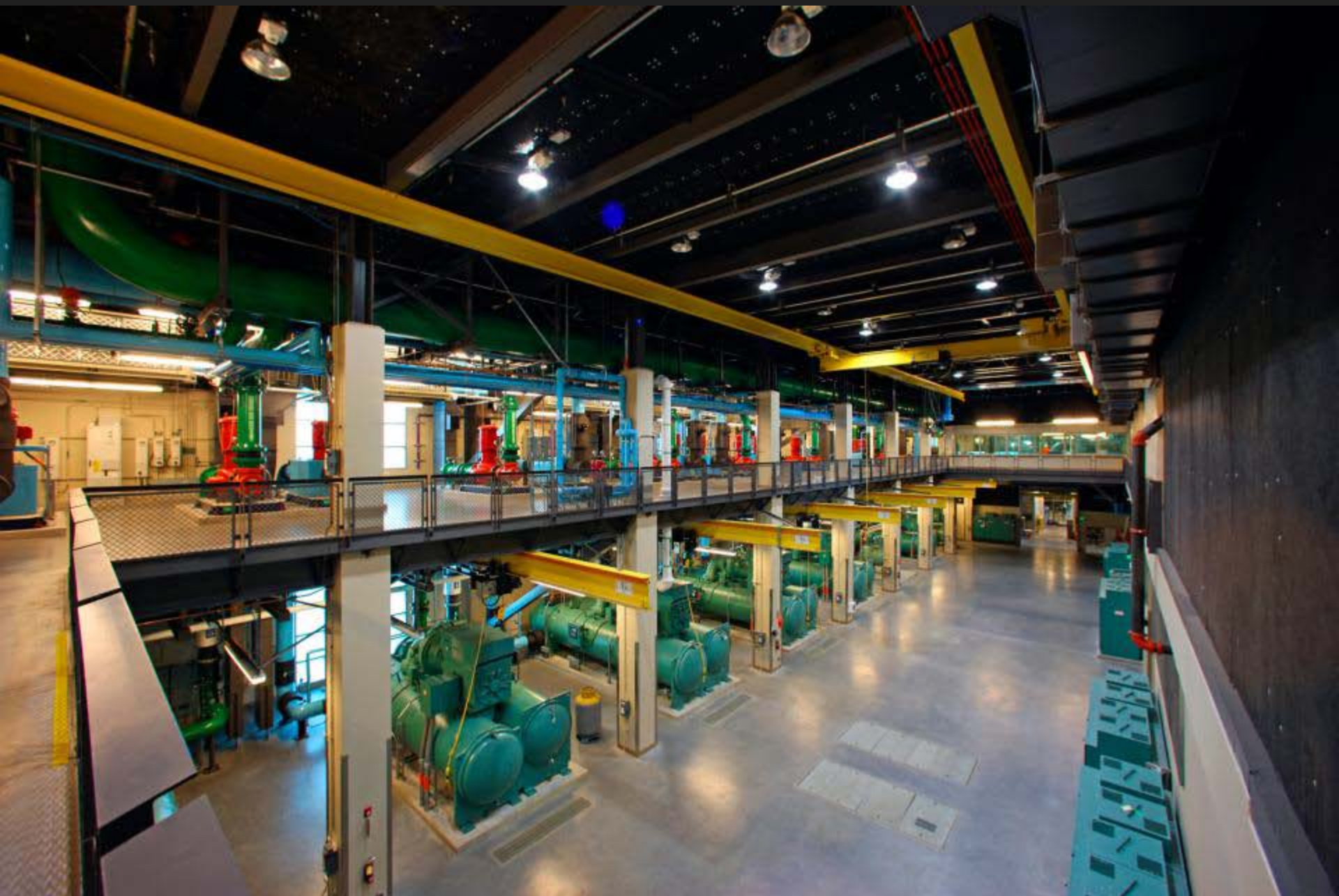
Chillers and VFD's at First Floor – Pumps and Control Room on Second Floor
