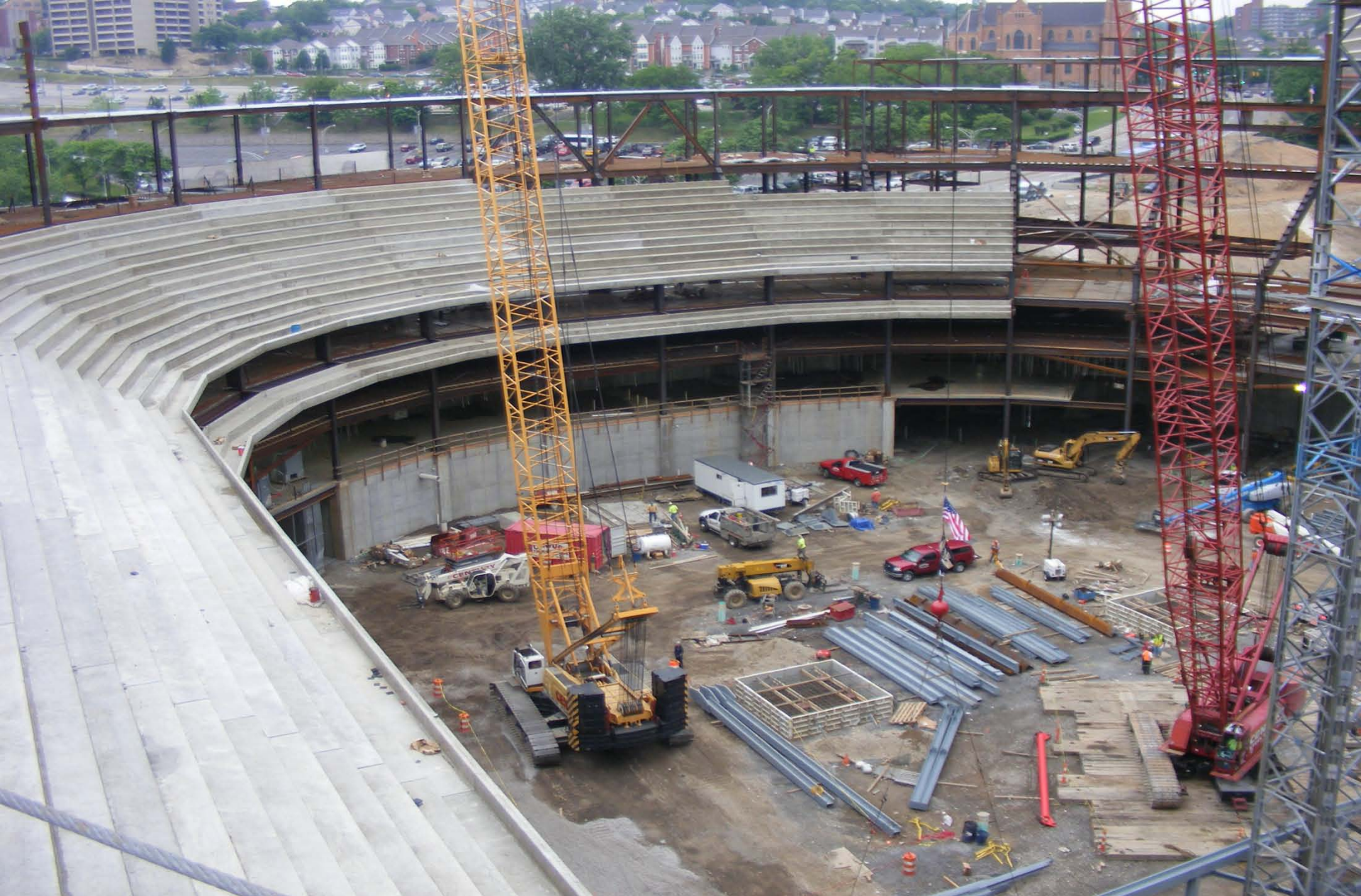
Upper down precast erection
