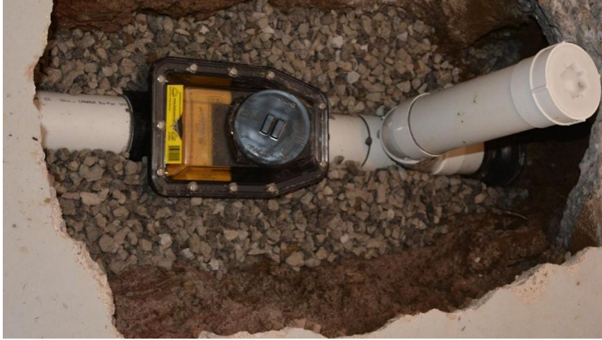
Figure C-3: A backwater valve during installation
