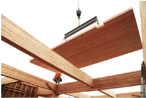
Building kits include prefabricated elements or sections that are then delivered and assembled on-site. The kit-of-parts approach, via panelization, is typical for mid-rise wood buildings. Image courtesy of LEVER Architecture
