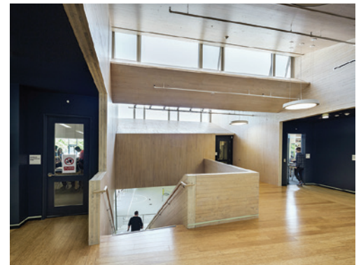
Black spruce CLT panels act as the tension surface and final ceiling finish in a revolutionary system of prefabricated stressed skin assemblies that span the upper classrooms and circulation spaces. Architecture: Gray Organschi | Photos: David Sundberg
