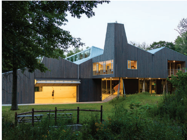
For the $7.5 million, Type VB, 15,000-square-foot addition, the project team chose a combination of CLT and glulam. The new school building was framed in just four weeks by a crew of five, using prefabricated materials. Architecture: Gray Organschi | Photos: David Sundberg
