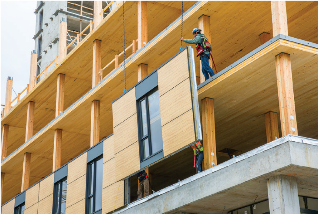
The foundation, ground floor, second-floor slab and stair/elevator cores are concrete, while the superstructure is composed of prefabricated cross-laminated timber panel floor assemblies supported on glue-laminated timber and parallel strand lumber columns with steel connections. Image courtesy of naturallywood.com
