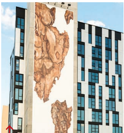
The playful façade of vertically oriented, reflective insulated metal panels, or IMPs, and window openings for a transit-oriented apartment building in Chicago carefully controls daylighting, thermal losses, and view corridors. The staggered windows create a sense of movement that is reflective of this fast-moving intersection, according to the project's architect, Wheeler Kearns Architects.
