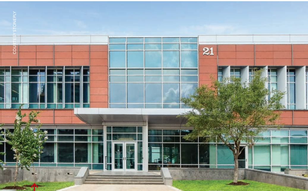
Thin-stone sandwich panels replaced the failing 1950s-era Georgia Pearl Gray marble slabs with matching quarter-inch cuts from the original quarry for the modern façade of the Arkansas Power and Light Building in Little Rock, now the headquarters of Entergy.
