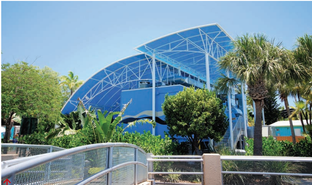
The Miami Seaquarium's exhibit for African penguins is a temperature-controlled volume made entirely of highly insulating structural magnesium-cement-board SIPs under a sun-blocking canopy.
