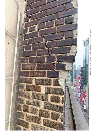
As maintenance is deferred, cracks and spalls proliferate into emergency hazards.
