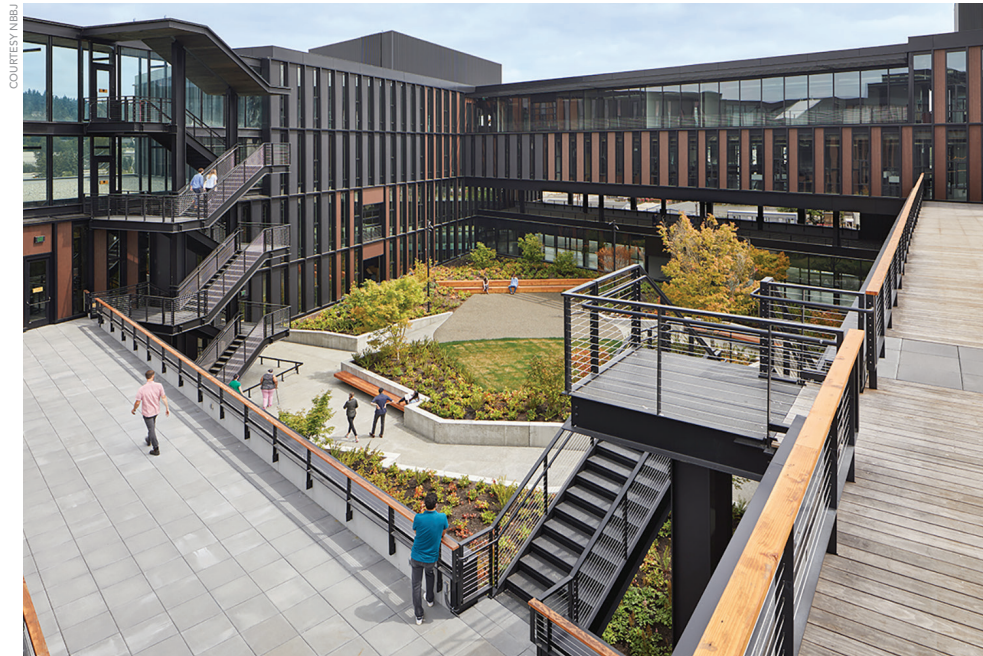
For an office campus for Meta’s Facebook in Bellevue, Wash., NBBJ and Turner Construction improved on the sprawling, eight-acre campus that expresses connection between work and nature. Originally designed for REI and then sold to Facebook, the newer Spring District building’s unique massing is clad with a custom-corrugated metal system in two finish tones: steel and bronze.
