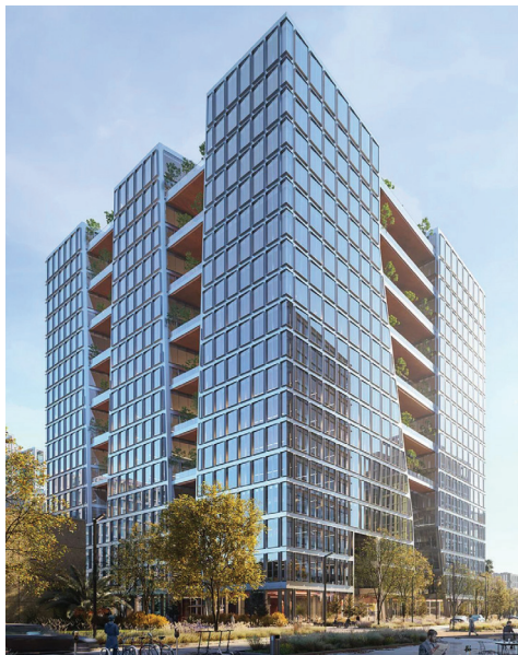
Clockwise from right: 200 Park, a 19-story office building in San Jose, Calif., employs a SpeedCore structural system. The system requires no temporary formwork for the typical concrete core. The basic structure is a concrete-filled, composite-plate shear wall system—two steel plates filled with high-strength concrete.
