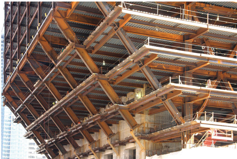
For 150 North Riverside in Chicago, high-strength steel formulations allowed for smaller, stronger sloping columns with fewer augmentations.
