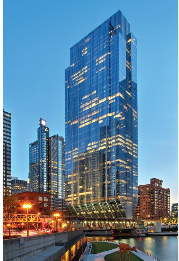
For 150 North Riverside in Chicago, high-strength steel formulations allowed for smaller, stronger sloping columns with fewer augmentations.
