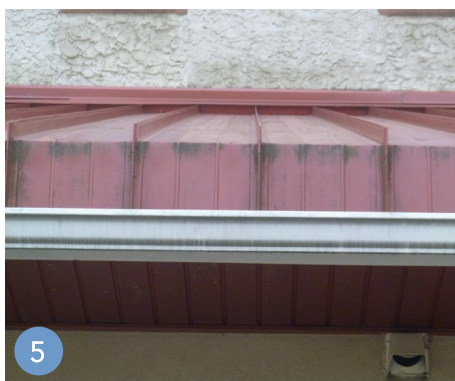
Common problems in metal panel systems include: 1) condensation, 2) corrosion, 3) movement and water intrusion, 4) peeling coatings, and 5) discoloration and staining.
