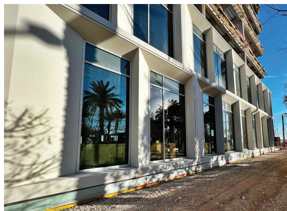
An innovative, light-colored cladding of preglazed, pre-insulated GFRC panels clads 1700 Pavilion in Summerlin, Nev., accelerating construction for the lifestyle-driven commercial building.
