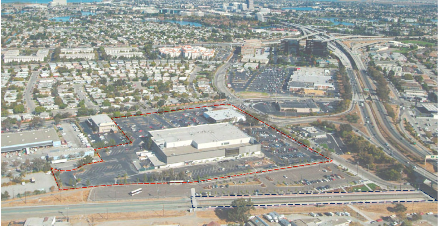
Top: Bird's eye view of the site conditions before redevelopment which included a Target, Michaels, gas station, and surface parking. (Credit - Google)
