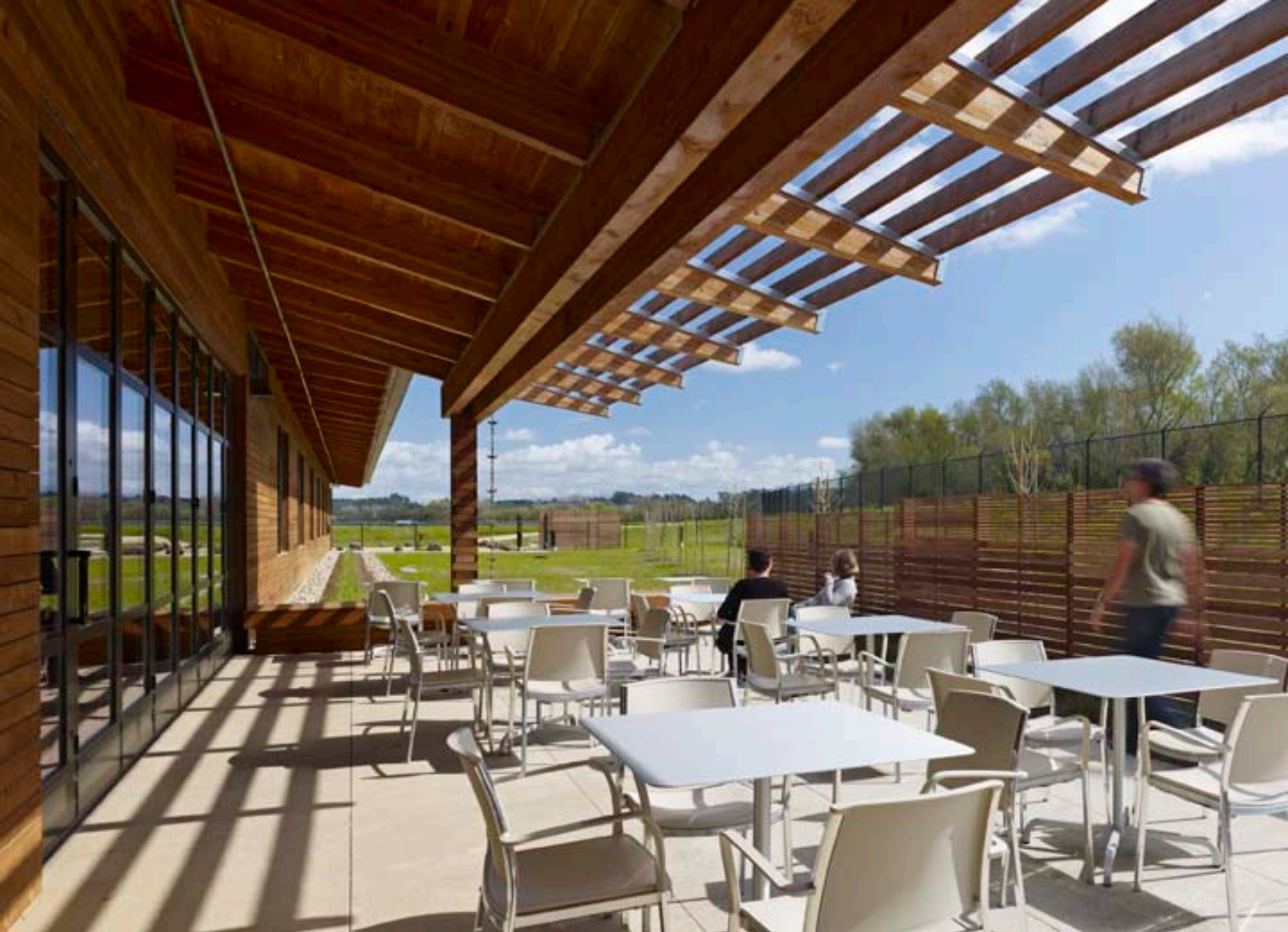
City of Watsonville, Water Resource Center Protected Outdoor Area
