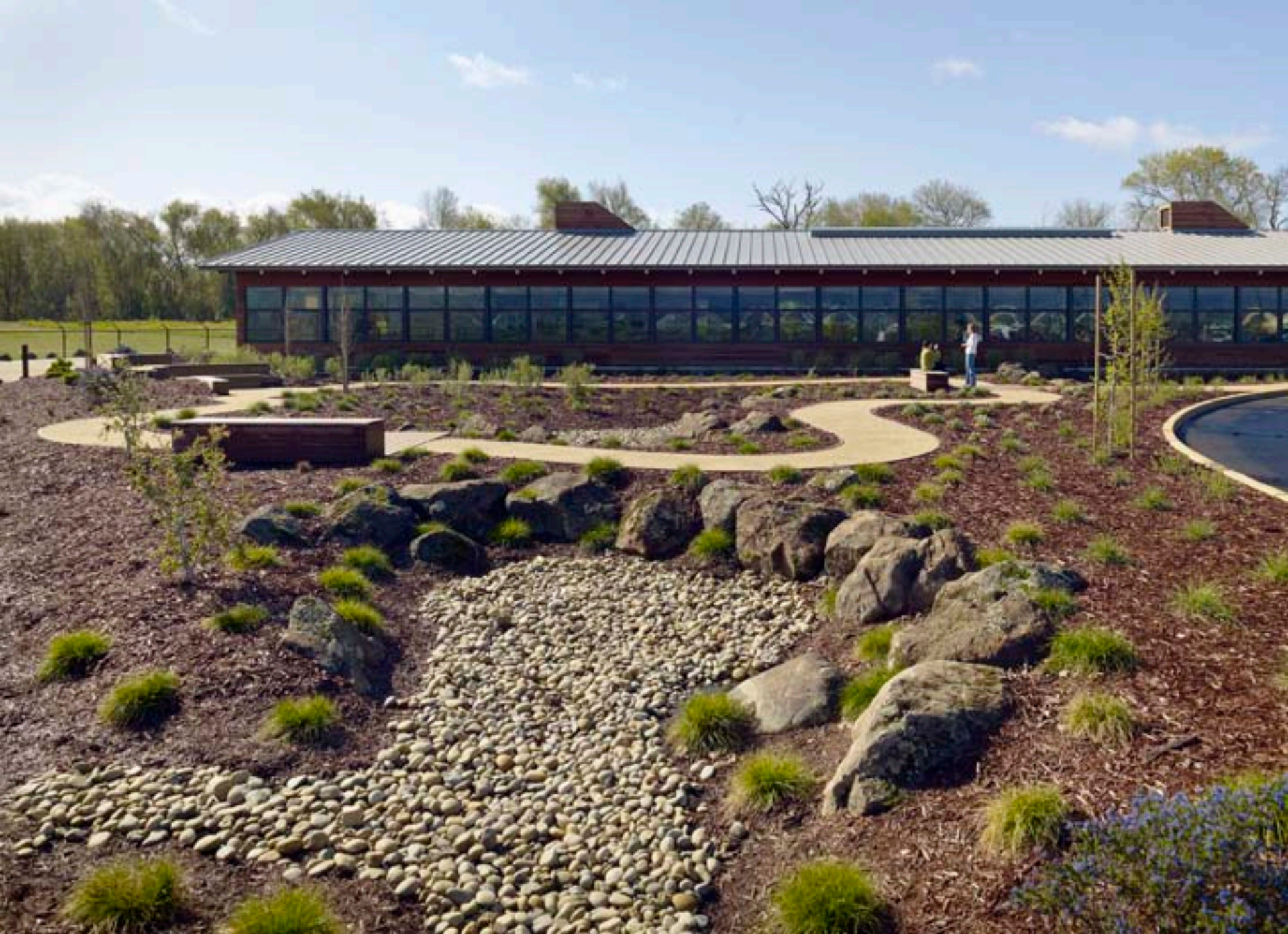
City of Watsonville, Water Resource Center Rock-Lined Bioswales
