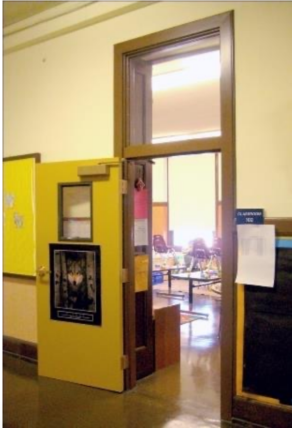
45 minute safety ceramic door lite and 45 minute non-safety ceramic in transom
