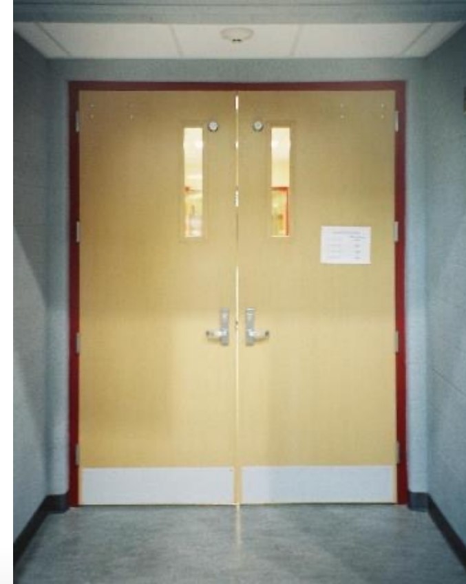
90 minute safety ceramic door lites limited to 100 square inches in 90 minute pair doors
