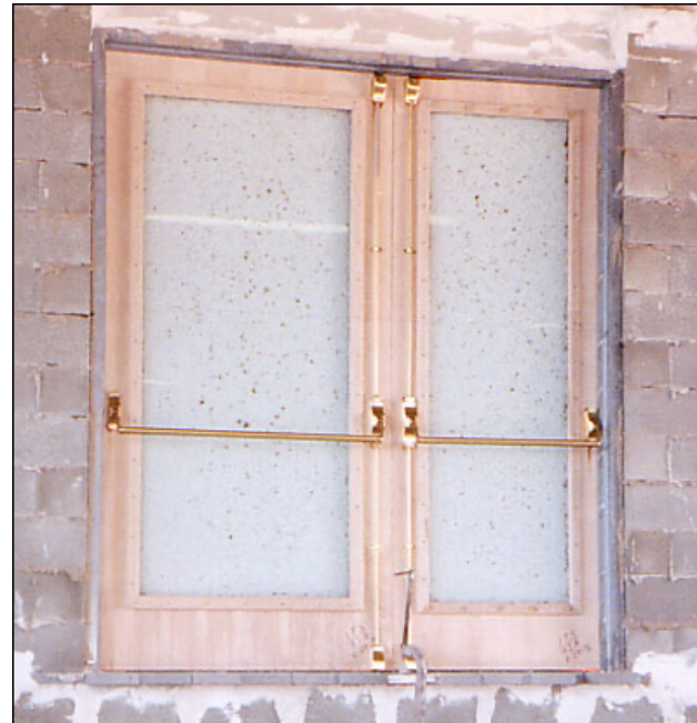
Fire retardant forms into absorbing char
