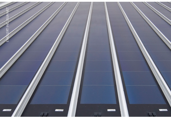
Left: Thin-film solar photovoltaics offer unique opportunities for integration with architectural metal roofs, and the solar cells are showing increased efficiencies and performance. Right: The ASTM E1592 Wind Uplift Test is recommended by FEMA and other groups over other testing methods to best represent a metal roofing system's uplift performance capability. The method evaluates the structural performance of sheet metal panels and anchor-to-panel roof attachments.
